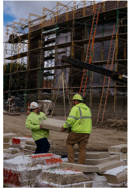
The school’s Mahan Hall is undergoing a renovation.
